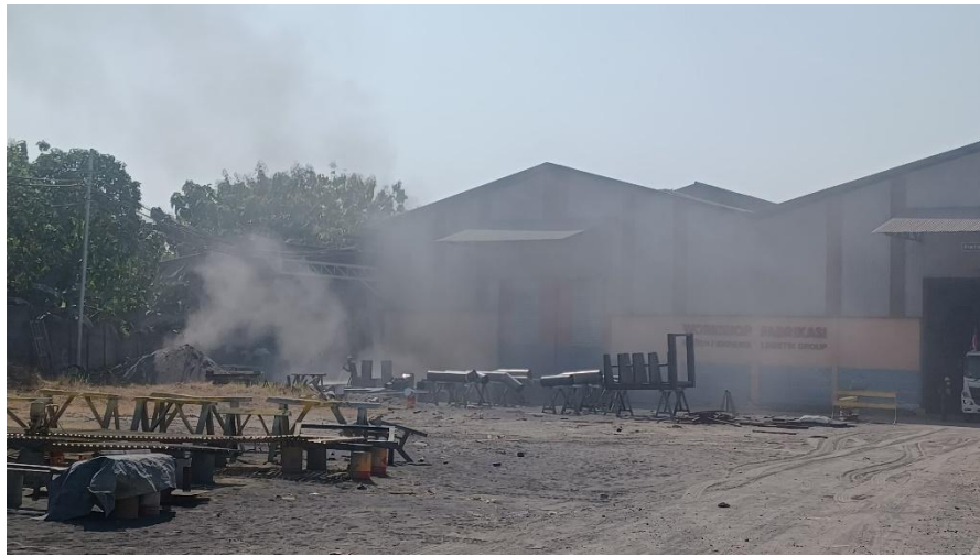
Gambar 1.2 Proses sandblasting area terbuka
